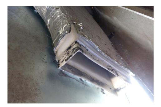
The upper wye is molded plastic, like the elbow that is attached to the heat pump, so it won't fail. It's the straight section between these two plastic pieces that comes apart. This straight section is made of ductboard which is attached to the upper wye with black mastic and 10 screws. The screws on the back of the duct are difficult. Don't pull the upper wye out too much or you'll tear the upper connections loose. A small right angle screwdriver worked for me.
