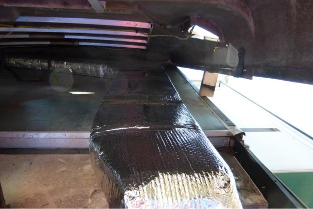
The finished installation. Plenty of insulation, which it did not have before. Just don't add too much insulation because it will affect the strapping of the duct to the wall of the coach and the alignment of the duct and plenums.
