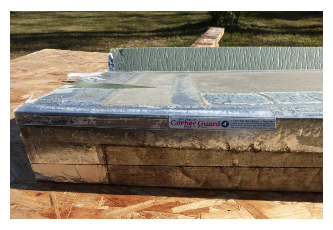
This is what is used to "reinforce" the corner joint. This photo shows the left over 12" piece that was randomly placed on one edge. The "Corner Guard" comes in 4' lengths and since the duct is only 36" long they have a 12" piece of scrap to discard, so they just stick it somewhere. This "Corner Guard" is a product intended to protect the corners of the interior walls of your house. It is not well suited to hold a duct together.
