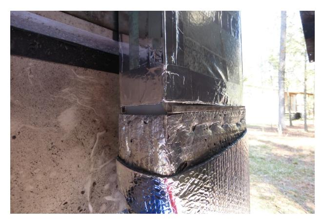
After I had the upper connection done and reinstalled the lower elbow plenum I saw that the lower connection was not square; about a ¾" gap at one end. This is the misalignment I mentioned earlier. I just used extra tape to cover the gap. I figure that if it fails it's at the bottom and can be easily reached. I did not use screws at this joint since it is basically held in place by compression.
