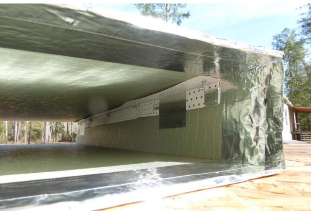
I used plastic drywall corner bead to hold the joint together. A piece on the inside and one on the outside with screws. It needs to be kept a few inches from the ends so it doesn't interfere with attachment to the plastic plenums.
