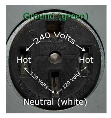
When you wire up a 14-50R 240V 50 amp outlet, you will measure 240 volts from hot to hot, 120 volts from each hot to neutral,
